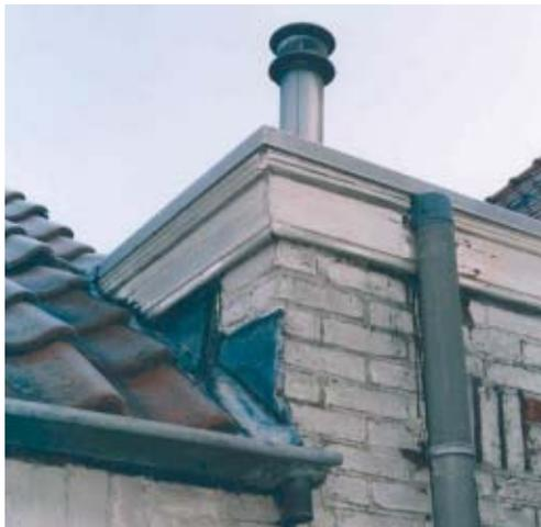
*Aluminium identified in roof strips and chimneys*
